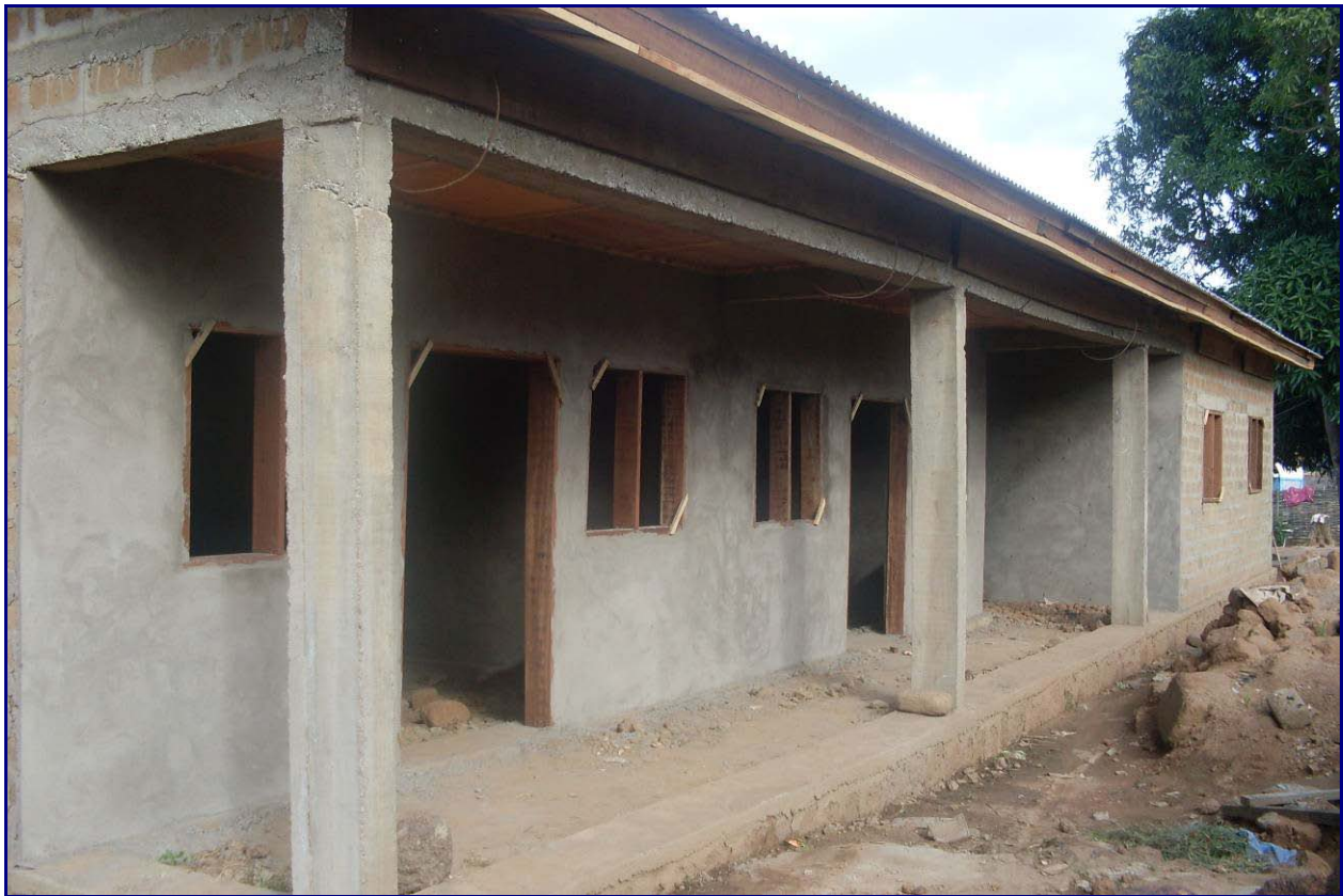
Interim stage of construction of the maternity ward
